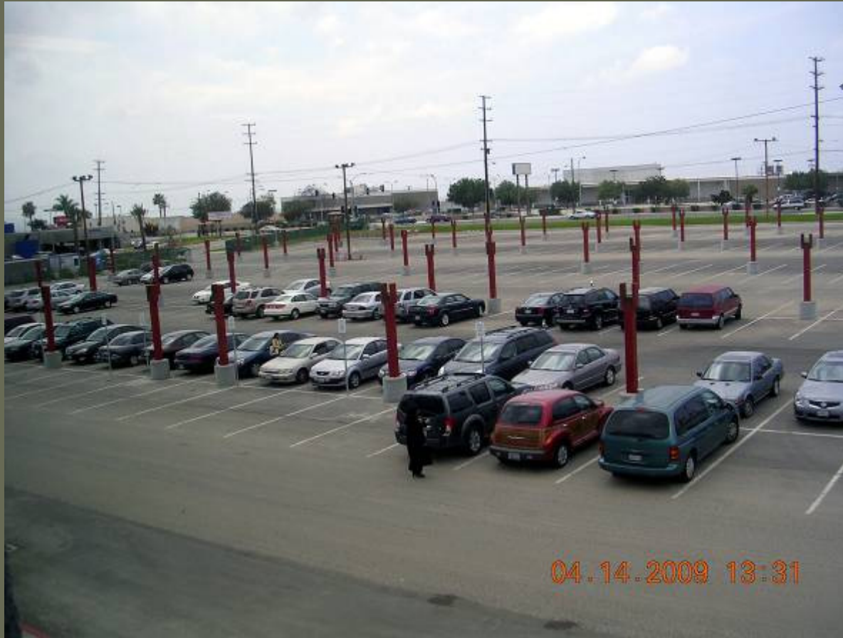
Lot 3 PV Installation
